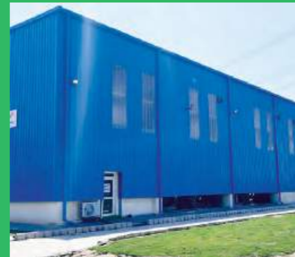
MVR LEACHATE TREATMENT PLANT, DELHI
