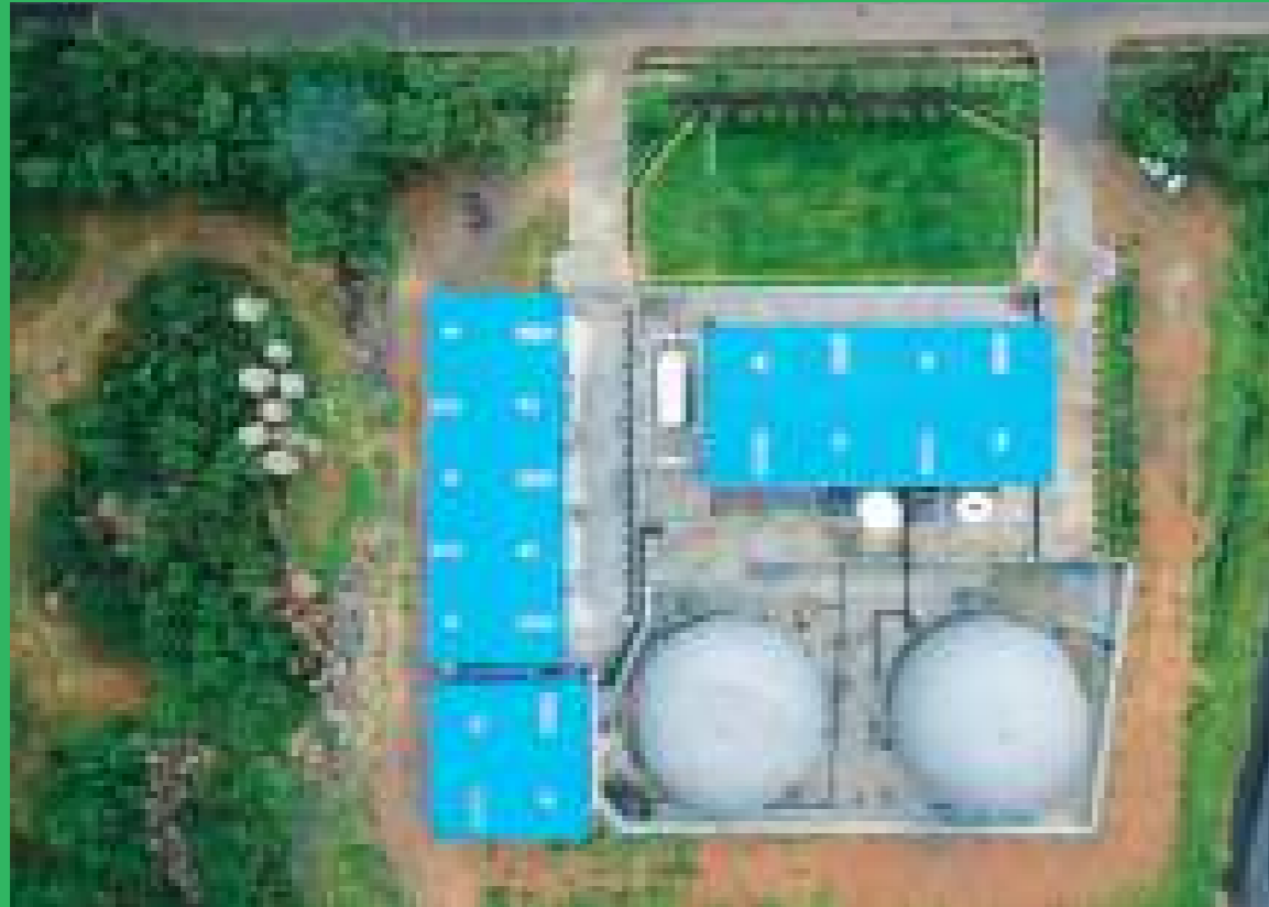
COMPRESSED BIOGAS PLANT, HYDERABAD
